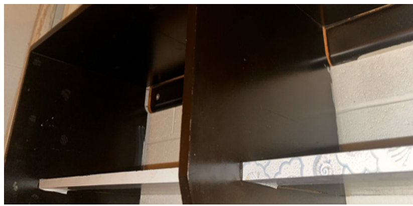
Photo credit Michelle Velez; Picture of broken closet shelf
