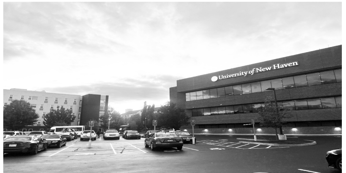
Parking lot that overlooks Celentano Hall and the library. Photo courtesy of Charger Bulletin/Azam Hostetter
